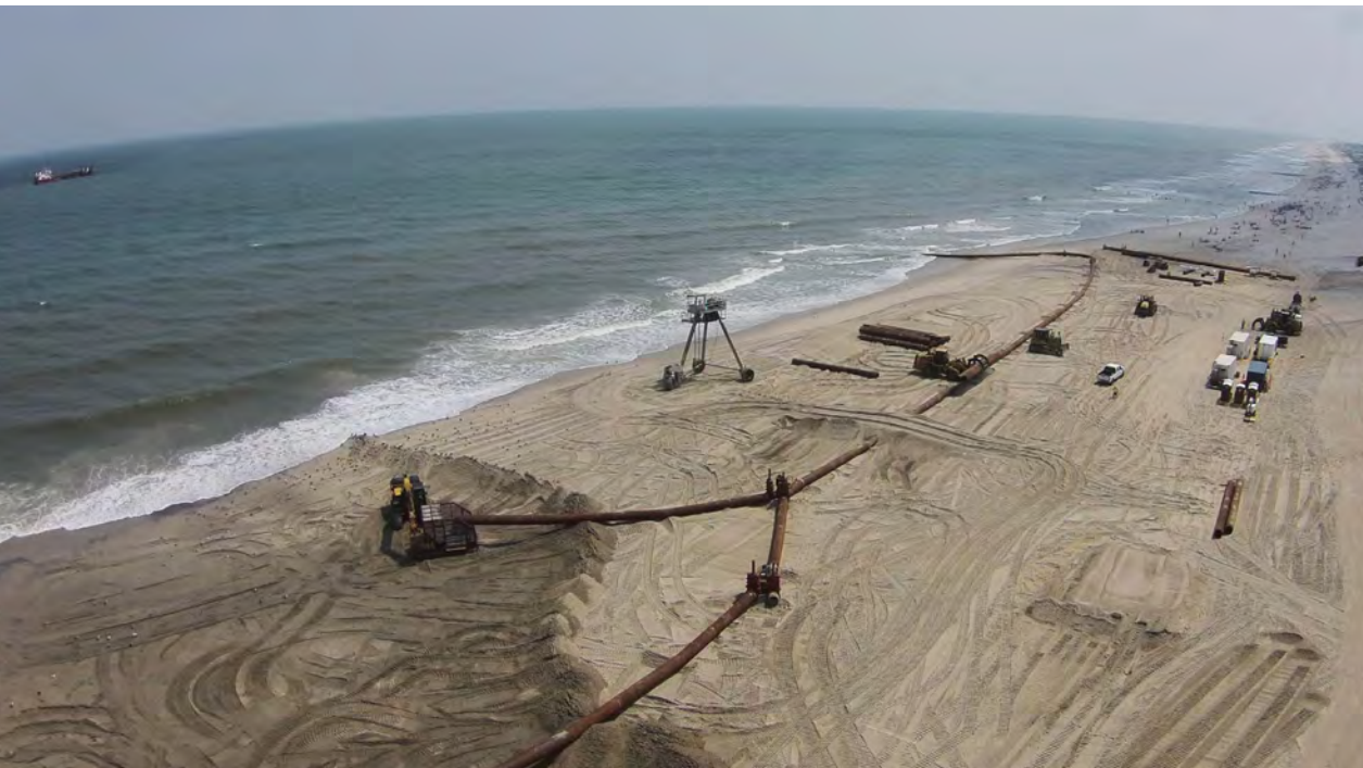
Aerial photograph of a beach nourishment project on Long Beach Island, New Jersey. © BOEM
