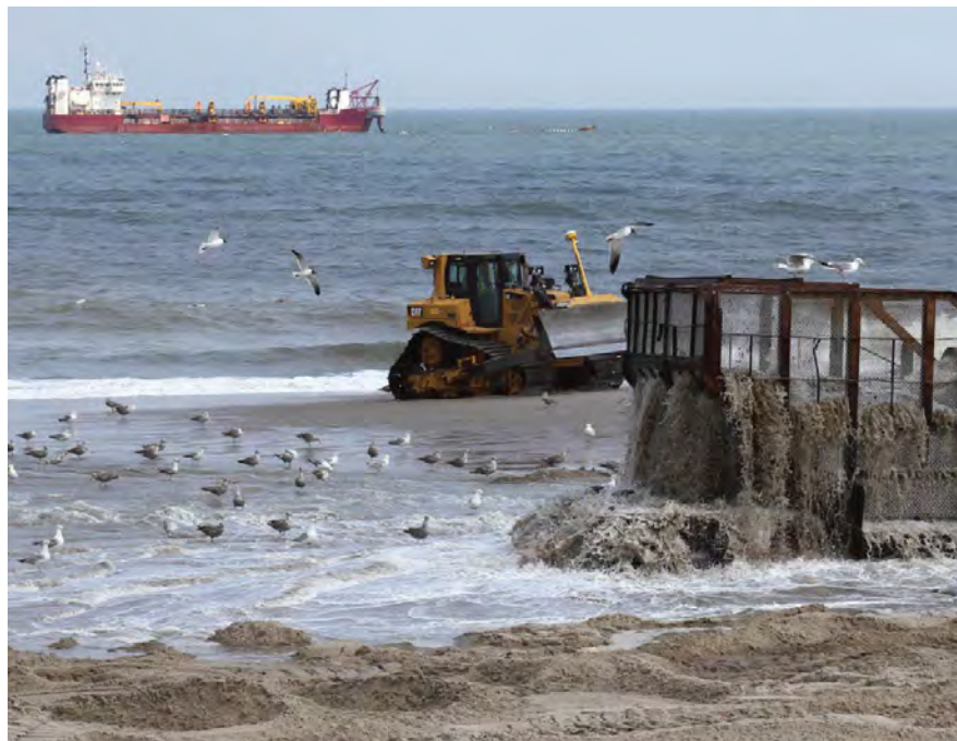
Discharge pipe with screen, construction equipment, and hopper dredge. © BOEM
