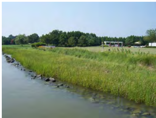
An example of a low sill living shoreline project in Maryland. (Photo: Bhaskaran Subramanian)
